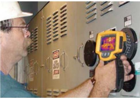
Example of a thermographer using an IR window and wearing standard level of PPE required while operating energized electrical equipment in an enclosed and guarded condition.
